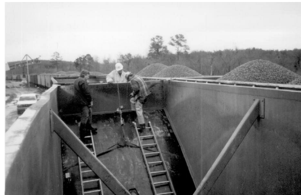
TIVAR® 88-2 end wall liner installation in progress.
